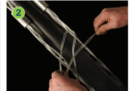
Thread the lace through the first two loops of the split and pull through until the laces are centered at this point.
