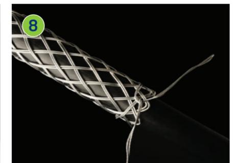
Add any additional support as required - banding is recommended. The cable grip is now ready to use.
